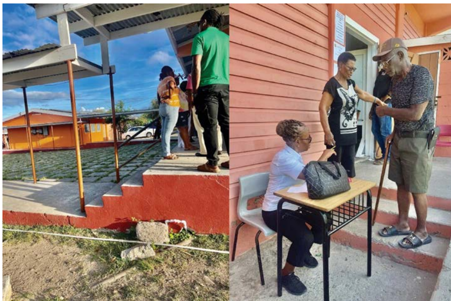
Figure 4.4 Some polling stations with stairs
