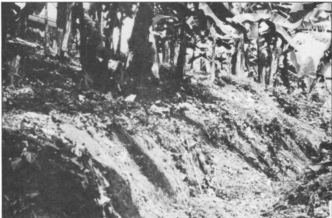
Figure 7.15 Eroded cutoff drain
